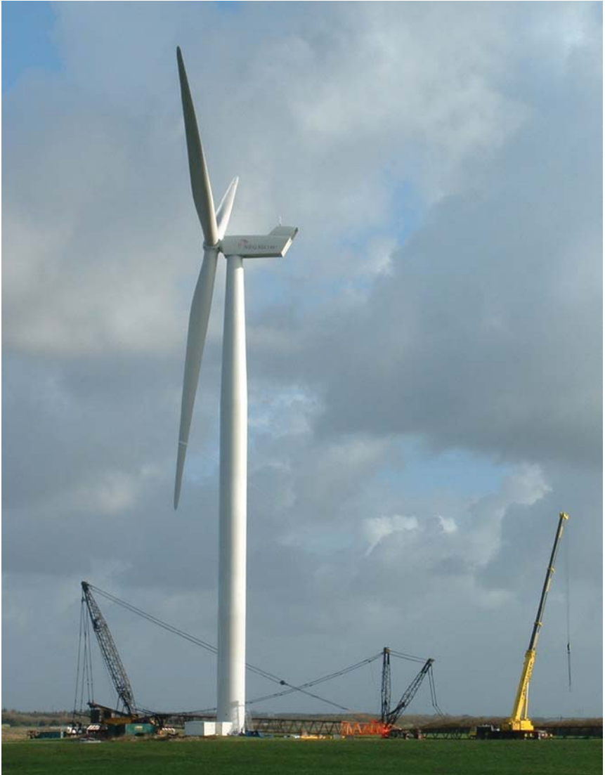
Figure 1 The world's largest wind turbine (summer 2004) at Risoe National Laboratory test site, Høvsøre, Denmark. Tower height is 120 m, rotor diameter is 110 m, and generator power is 3.6 MW.
